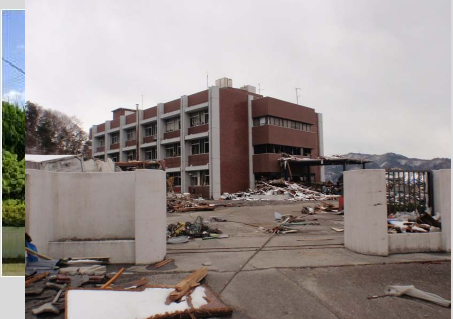
Main building of ICRC in Otsuchi Town before and after the tsunami on Mar 11
